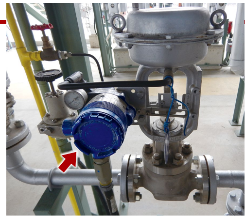
HART communication between the smart valve positioner attached to the valve and the device management system allows the operating status of field equipment to be visualized.
