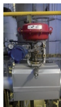
Sending control valve operation data to the cloud to formulate control valve maintenance plans with CBM
