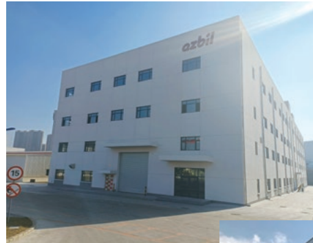
The new factory building in Dalian, China, which has begun operation. An advanced control valve production system is under construction.
