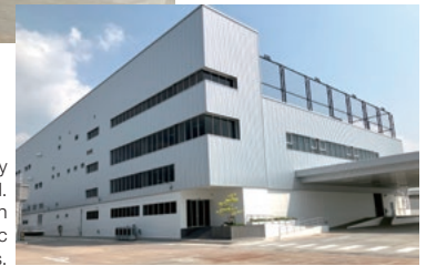
The newly completed factory in Thailand. We plan to build production lines for electromagnetic flowmeters and other products.
